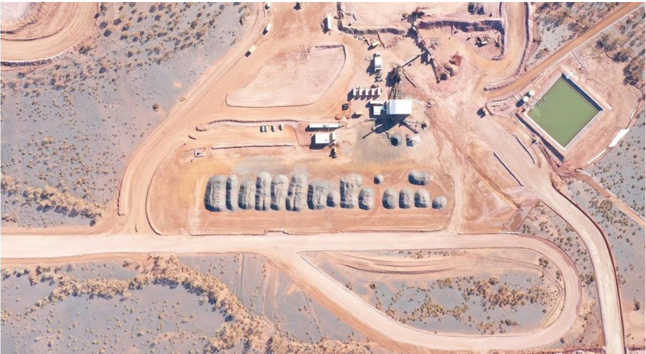
Figure 1 - E25's completed Stage 1 operation at the Butcherbird mine site in Western Australia
