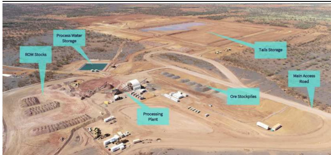
Figure 7: Processing plant and infrastructure at Butcherbird
