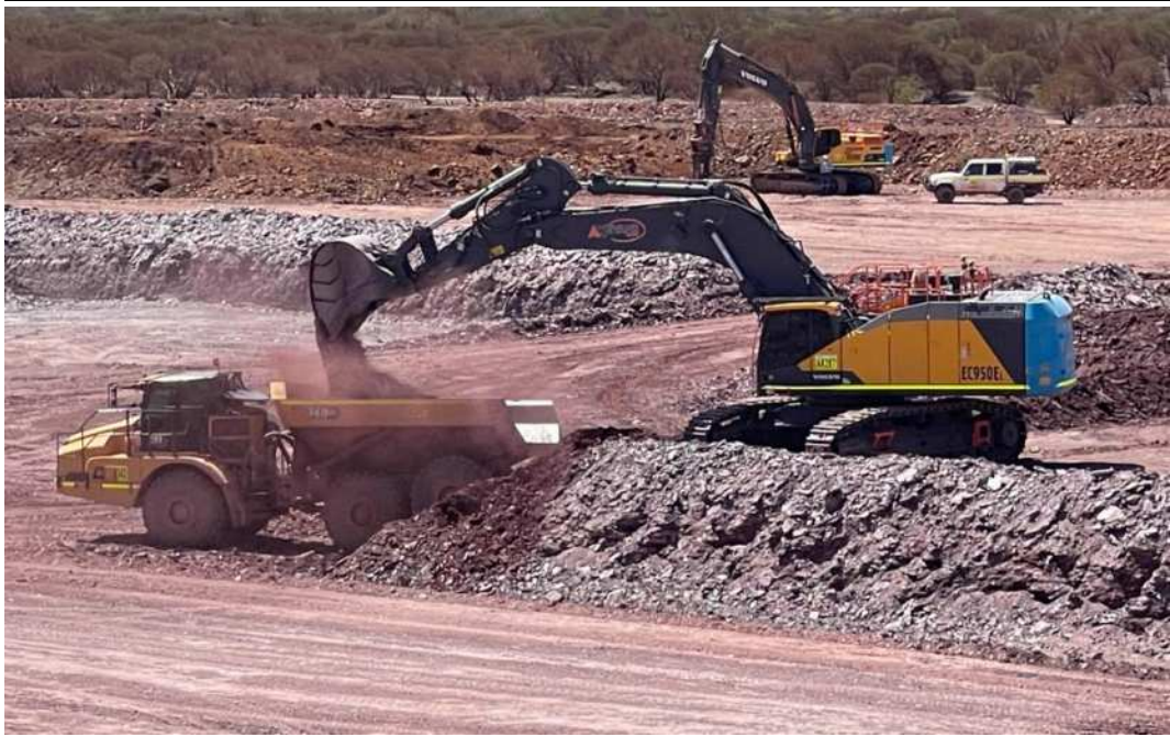
Figure 5: A dozer and excavator working on site
